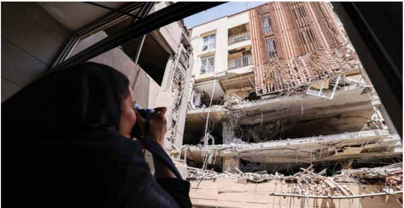
A photojournalist captures a damaged residential building hit by an Israeli strike in Tehran on June 25, 2025. ATTA KENARE/GETTY IMAGES
